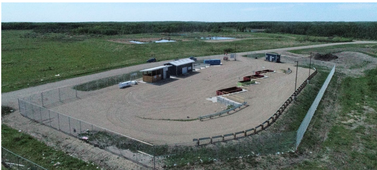
Figure 3: Ochapowace Nation Transfer Station
